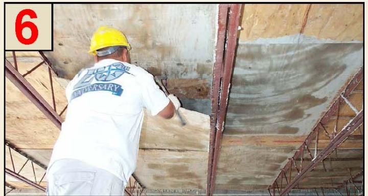
**Stripping the Formwork:** Rollbars and plywood are stripped, usually the day after the pour or once the concrete reaches 500 psi. The deck is ready for other trades when the concrete reaches a strength of 1,000 psi.
