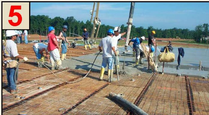
**Pouring Concrete:** Minimum 2-3/4" 3,000 psi monolithic slab forms an acoustical seal where the slab passes over walls. The top chord protrudes into the slab for composite action, and serves as a guide for screeding.
