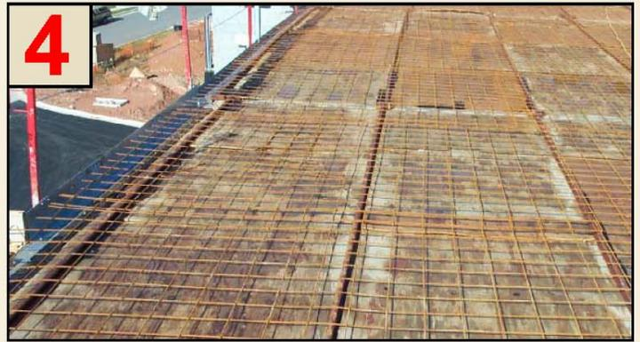
**Mesh in Place:** Standard 8' x 20' sheets of mesh are easily placed over top chords of Hambro joists. The mesh drapes and forms a natural catenary to reinforce and support the concrete slab.
