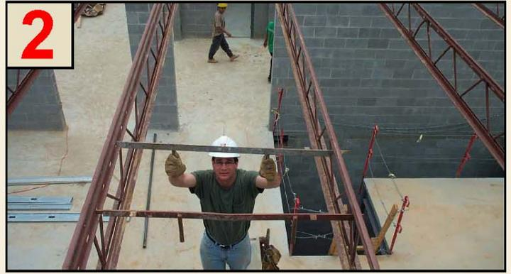
**Placing Rollbars®:** These secondary members support the forms, slab and construction loads. Rotated and locked into holes in the top chord, Rollbars guarantee exact joist spacing while providing lateral and torsional stability. Typically, no permanent bridging or bracing is required. Bottom chords are fabricated with clips to accommodate a Rollbar for additional bracing as required.
