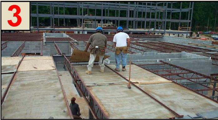
**Installing Plywood Forms:** The system reuses full sheets of standard 3/8" CDX grade plywood. Plywood is lapped and together with the Rollbars provides a secure platform during construction. Where 1/2" or 5/8" plywood is used, no lapping is permitted.
