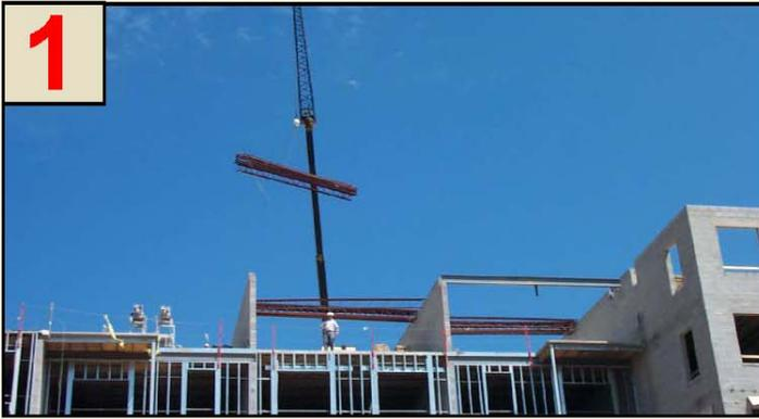
**Spreading the Joists:** Bundles of joists are placed on walls or beams and spread to approximately 4' o/c. With this greater joist spacing, the number of joists to be handled is reduced - a benefit in joist sorting especially on tight sites where space is limited.
